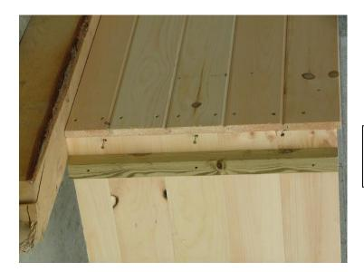
The lid is screwed into the back wall using seven to eight 1-5/8" zinc screws along the top of the back wall.
