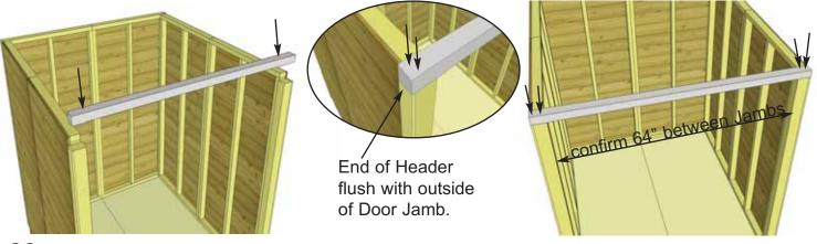
**23.** Position and attach the Door Header flush to outside end of Door Jamb with 2 - 2 1/2" screws per side. Important- Drill 1/8" pilot holes in end of Door Header to prevent wood from splitting.
