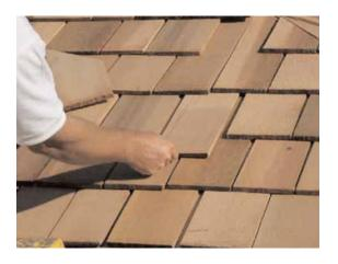
**41.** Slide in another Long Filler Shingle and attach as per **Step 40.** On your last Filler Shingle, attach to roof with 2 - 1 1/4" finishing nails.
