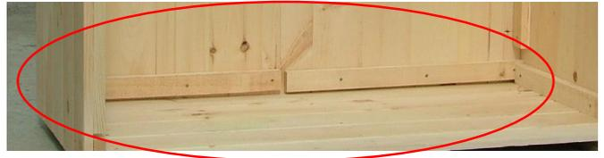
Front is attached using two 1-5/8" Zinc screws each side.
